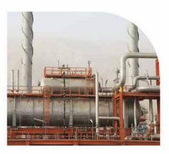
The deaerators can bring down the oxygen content of the boiler's feed water to 7ppb ASME, ASTM, and HEI standards are used in designing and construction of these products.
