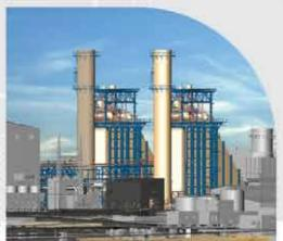
Incase of gasturbine out aged ue to maintenance, our HRSGs can take the advantage of Fresh Air Firing system, consisting of air fan and burner in general, when the steam generators can keep producing steam independent of GT ,called Stand-Alone operation.
