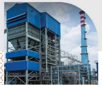
Sometimes the exhaust gas of industrial processes carry suspended particles and different pollutants, in this situation, WHRB packages are equipped with online cleaning systems, and various requirements are considered in the design of their thermal surfaces and the materials used.
